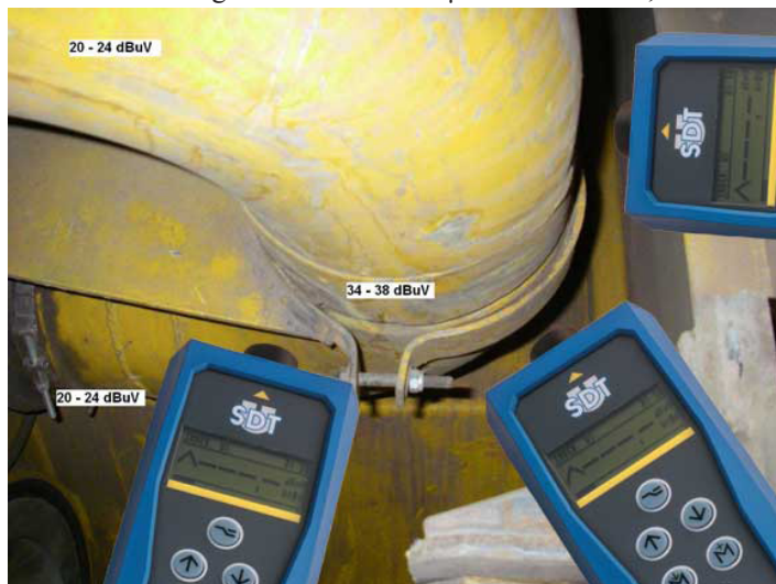
Image 8 - Scan the breather system from filters to turbo charger with SDT170
